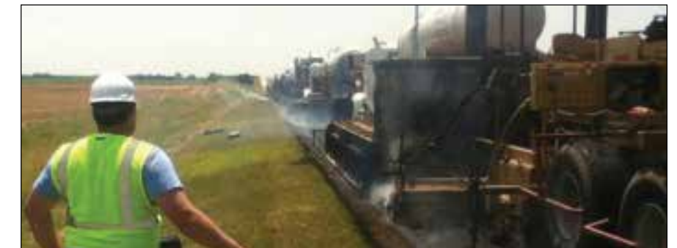
Doctoral candidate, Brandon Bortz, waits to sample materials as the HIR train heats, scratches, breaks and replaces old asphalt pavement on K-14 with a new layer.
