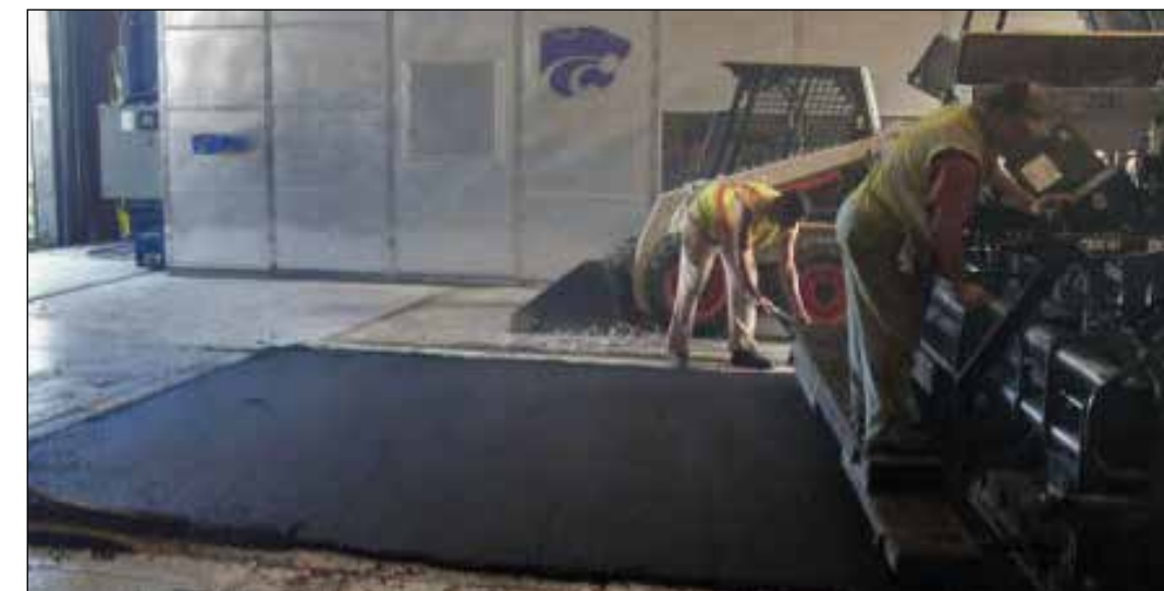
Test sections being paved at CISL to test the bond between asphalt layers
