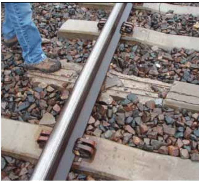
CE researchers inspect concrete tie failure in track (inadequate bond is believed to be one of the primary causes).
