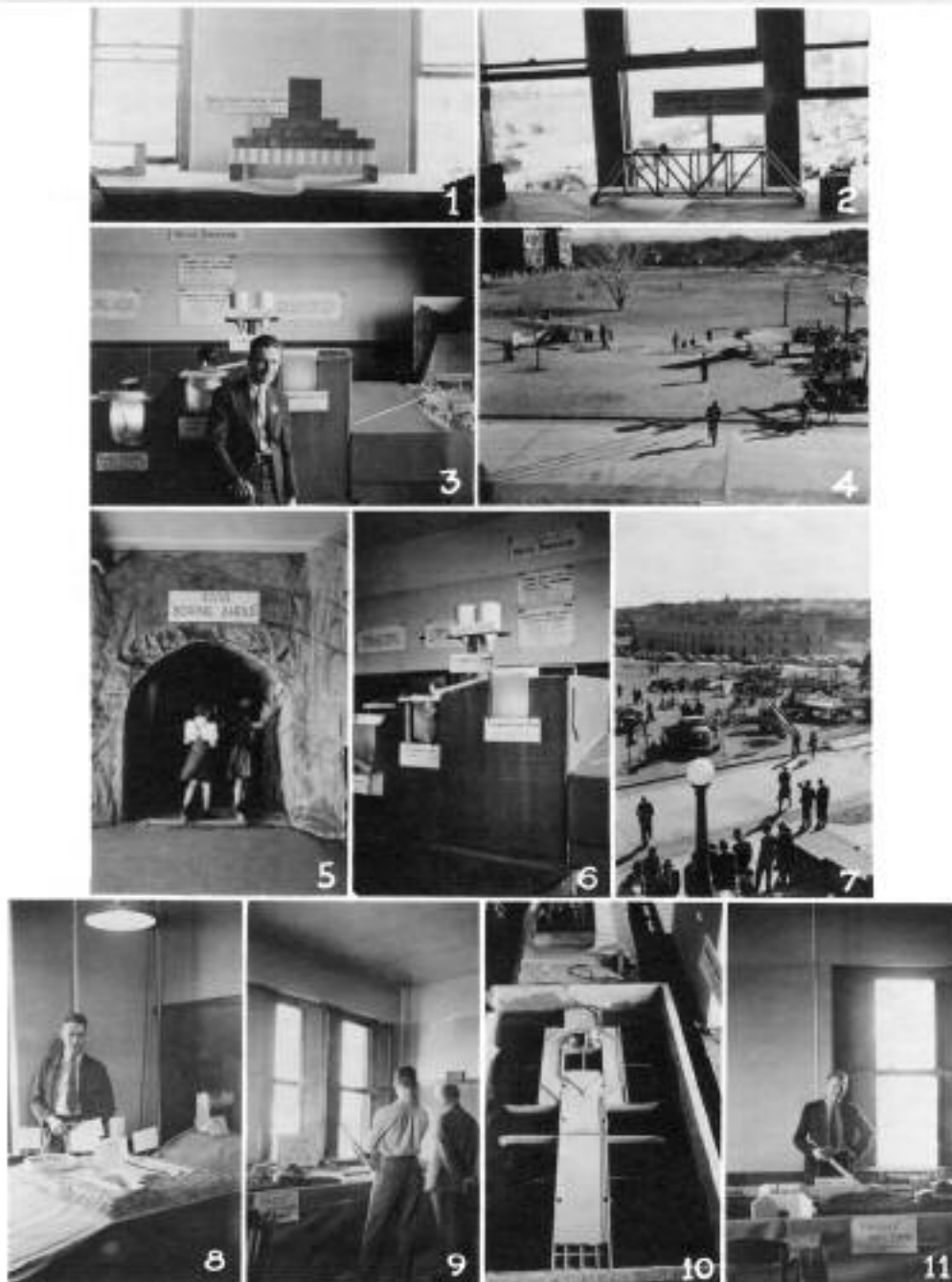
(1) A plate girder deck railway bridge constructed of paper and loaded with 104 pounds of bricks. (2) A model of the Warren Truss demonstrated the principle of the reversal of stresses in web members as a load passed across the structure. (3) Working model of a water purification plant. (4) Model airplanes on display at the 1940 K-State Open House. Picture taken from Seaton Hall. Note Kedzie Hall in the background. (5) "Civils Boring Ahead" display. (6) Another view of the water purification plant model. (7) More displays. Picture taken from Seaton Hall. Note Memorial Stadium in the background. (8) Working model of a "modern" sewerage treatment plant. (9) Room-length model of "modern" highway construction from the preliminary survey to putting the finishing touches on the concrete slab. (10) Model of a floating bridge then under construction over Lake Washington. (11) Another view of the highway construction model.
